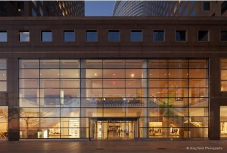
In the south, the glass fins allow an almost unobstructed view to the interior of the building and outside. Photo: Greg West Photography
