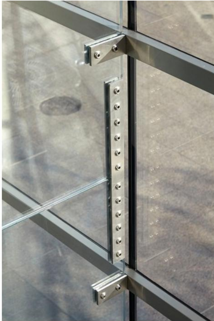
The 7m long glass fins bear the load of the all-glass façade. The connection parts are kept unobtrusive so that the transparency of the building envelope is hardly affected. Photo: Greg West Photography
