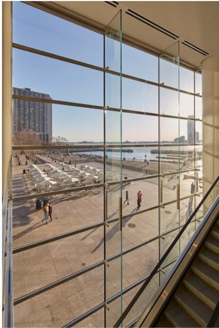
The façade elements are connected to 7m long glass fins. Thus, the view of the Hudson River is nearly undisturbed. Photo: Greg West Photography
