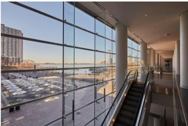
The transparency of the all-glass façade creates openness and allows an unobstructed view of the Hudson River. Disturbing metal constructions are unnecessary thanks to the 7m long glass suspension systems. Photo: Greg West Photography
