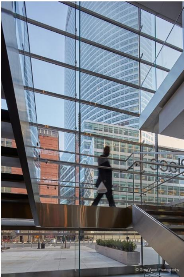
Thanks to the large size glass fins, the façade elements only need few connection parts making the building envelope highly transparent. Photo: Greg West Photography
