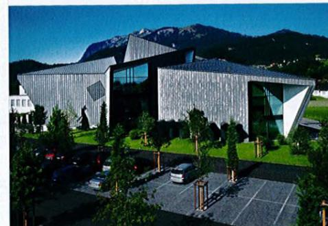
The steel section system VISS SG from Jansen AG was inserted into the glass façade, allowing large openings within the façade. VISS SG is Jansen's system for structural glazing façades (Copyright: Jansen AG)
