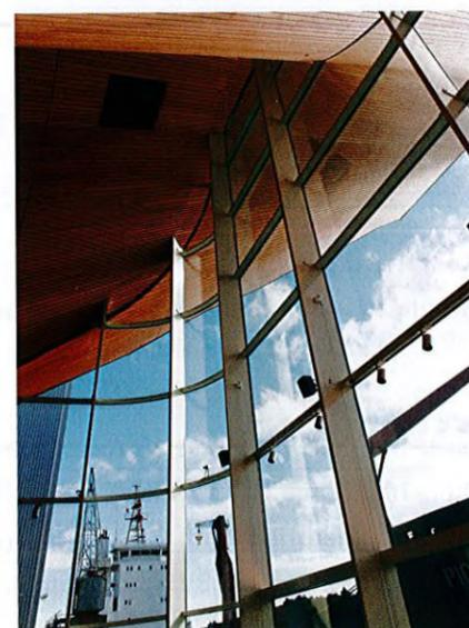
The panoramic façade, bent at the edges, penetrates the curved roof design. It was realised with Jansen VISS Ixtra high-precision, laser-welded steel sections. (Image copyrights: Jansen AG)
