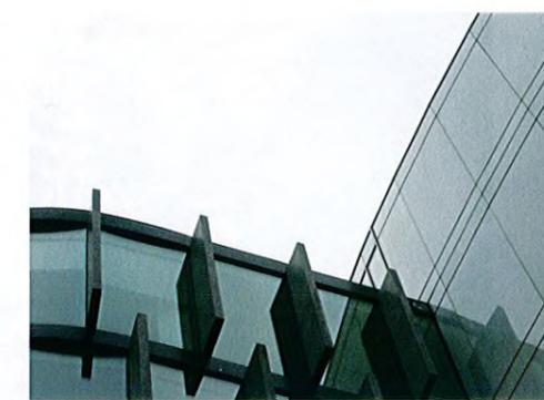
Example of a structural glass façade with visually "penetrating" concrete elements (Copyright: Rainer Hardtke)
