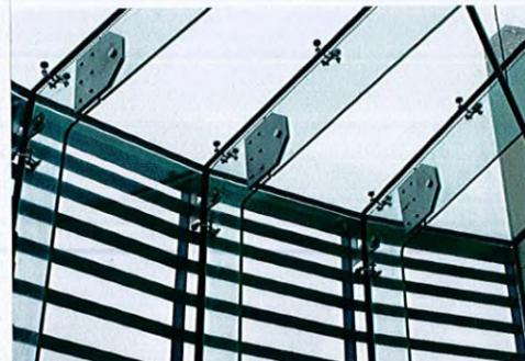
Interior of a spot-fitted façade with load-bearing glass support (Copyright: Rainer Hardtke)
