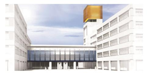
Two characteristic elements and the material glass make the new building of Cambridge Assessment a landmark. Together with the tower, the backlit glass façade out of orange-colored laminates form an architectural accent that is visible for miles around. The blue printed IGUs of the Skywalk link two wings and are a visual counterpart of the tower.
